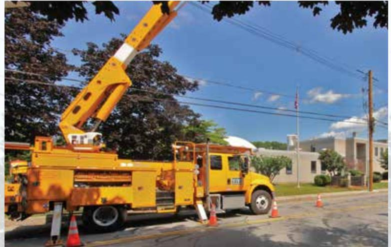
LELD crews have been on site on Harvard Road replacing poles and upgrading infrastructure to meet the electrical demands of the new Patriot Beverages, which has notified LELWD of its intentions to reopen the bottling plant for full-scale production near the end of 2018 or beginning of 2019.
